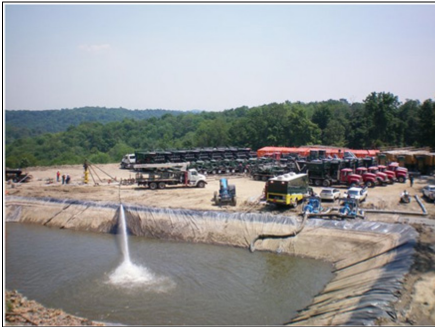
Figure 11. Temporary storage pond used in hydraulic fracturing
