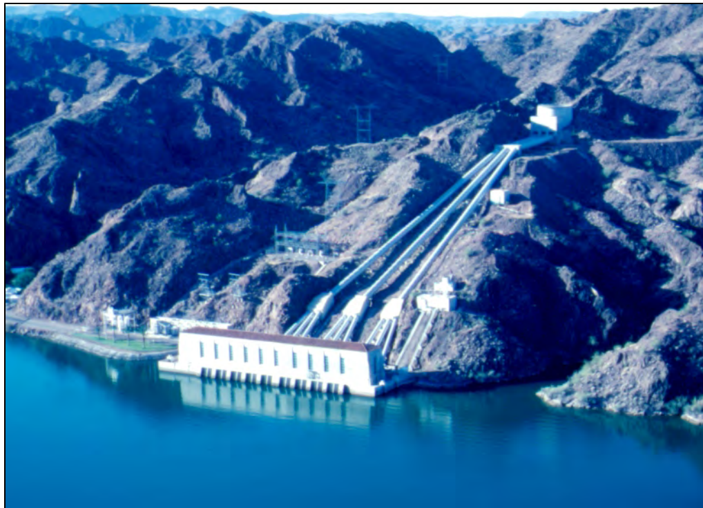
Figure 3. Metropolitan's Whitsett Intake Plant. The plant pumps water from Lake Havasu to the Colorado River Aqueduct, 49 for distribution to 23 of Metropolitan's 26 member agencies. 50 Source: The Metropolitan Water District of Southern California
