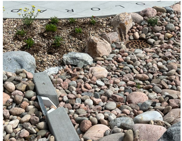
Stormwater monitoring weir and drain at the CSU Spur Campus. Source: Jane Clary
