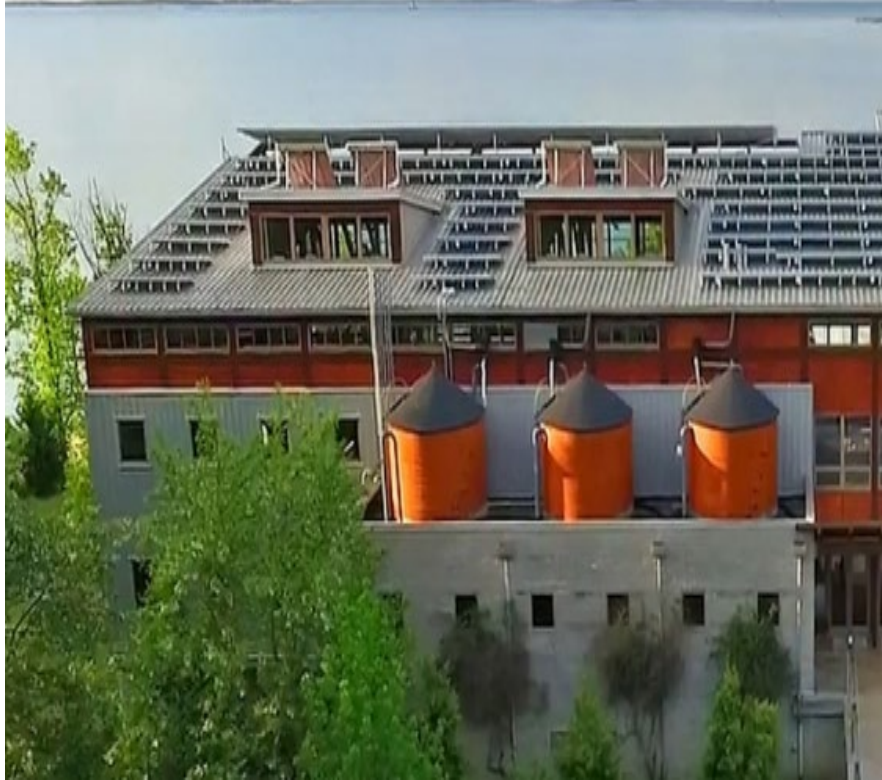
Figure 2. Rainwater is captured, treated, and used for fire suppression and other activities at the Philip Merrill Environmental Center, headquarters for the Chesapeake Bay Foundation and a LEED Version 1 Platinum certified building. Photo by DroneVideoNow.
