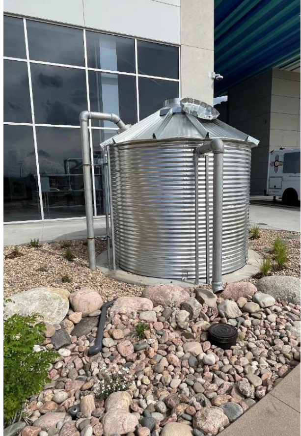
Photo 2. Cistern at the CSU Spur Campus. Source: Jane Clary
