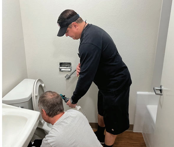
The installation of the leak sensors. ©Cora Snyder, Pacific Institute.
