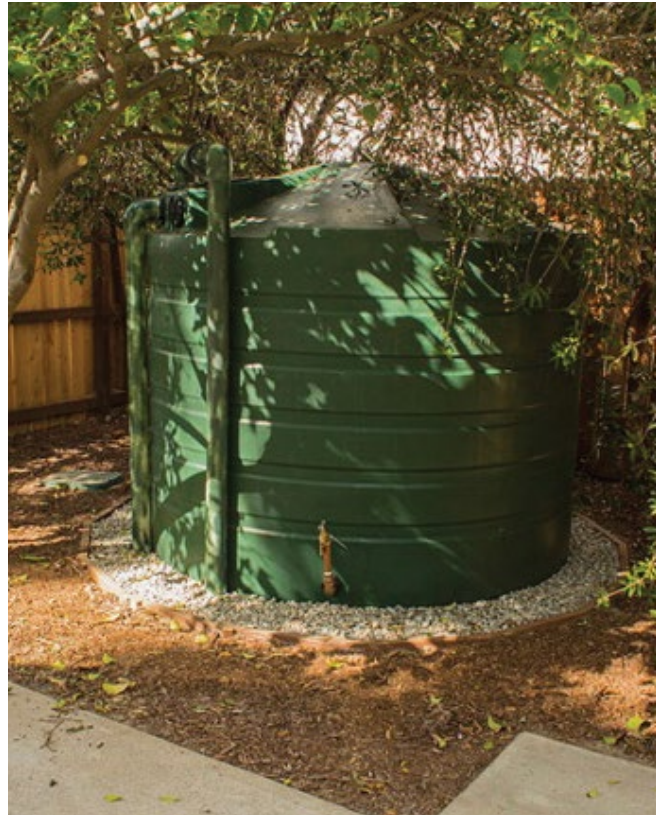
Rainwater harvesting system in Los Angeles, California.
