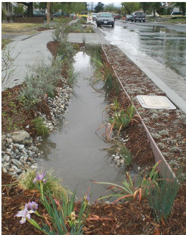
Bioswale on Elmer Avenue in Los Angeles, California.
