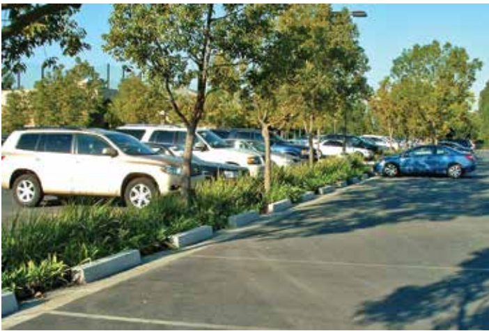
A vegetated swale in a parking lot © Haan-Fawn Chou
