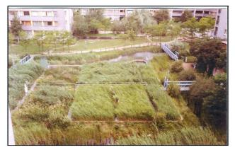
Figure 5. Constructed wetlands used to treat greywater from a housing development in Berlin, Germany. Source: Nolde Grey Water Recycling
