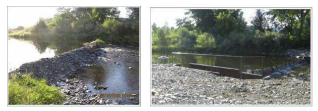
Figure 21 Before: A gravel and wood "push-up" dam that blocks fish passage on the upper mainstem John Day River, south of John Day... And after! The lay-flat stanchion dam includes a channel for fish to migrate past the dam. When the dam is lowered, the stream flows naturally (photos and caption from BPA 2009).
