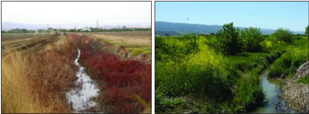
Figure 3. Willow Slough on Oakdale Ranch before the project (left, an incised drainage ditch with steep banks covered in non-native vegetation) and after (right, more gently sloped banks provide a lower bench for high floods covered in native grasses and an upper bench with a maturing riparian forest).
