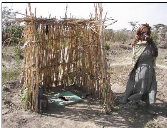
Figure 16. Arborloo built by Catholic Relief Services Photo credit: Catholic Relief Services
