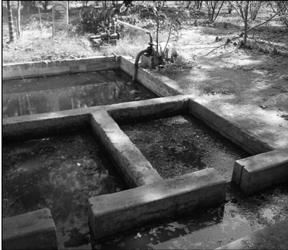
Figure 9. Wastewater collection pond used for irrigation in Kikware, India
