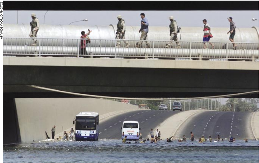
U.S. troops in Iraq August 2003 inspect a water pipe damaged when an explosion tore a hole in it. Water systems have continued to be the targets of insurgents fighting the U.S. invasion.
