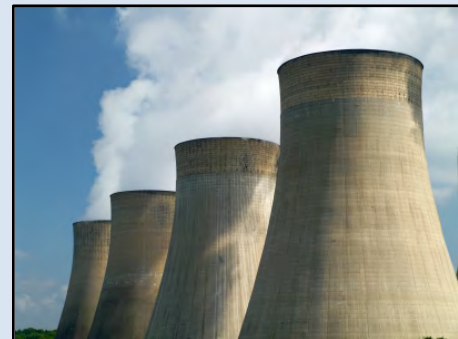
Figure 6. Photo of wet cooling tower
