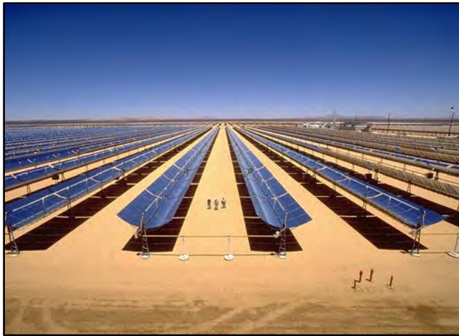
Figure 3. Solar photovoltaic system in New Mexico Source: Worklife Siemens/Flickr.com
