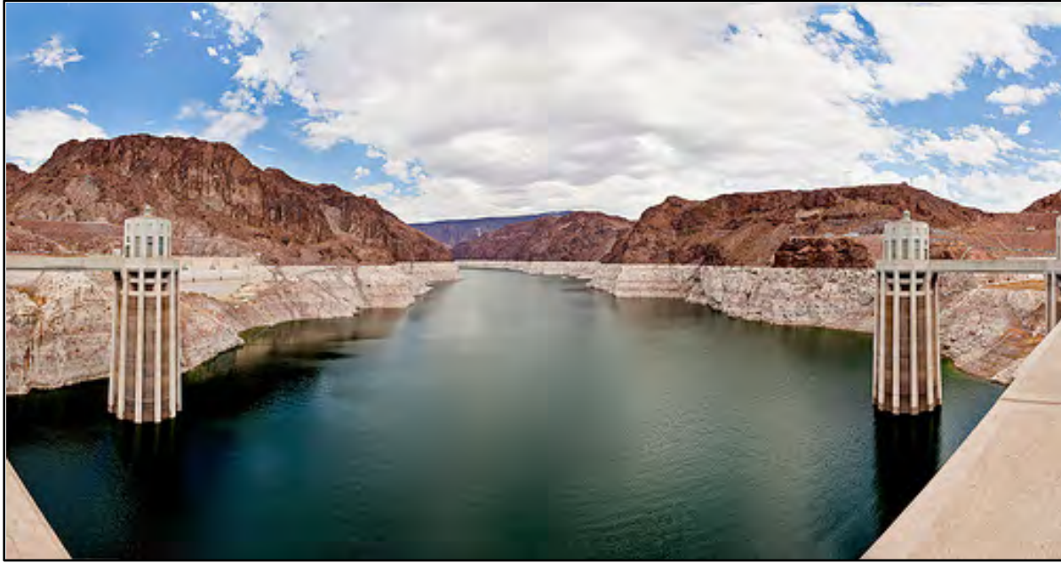
Figure 17. Low water levels in Lake Mead threaten hydropower generation
