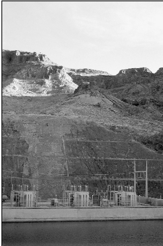
CAP intake at Lake Havasu. CAP water is lifted nearly a thousand meters in elevation before reaching its terminus south of Tucson. (Photo by J. Morrison)
