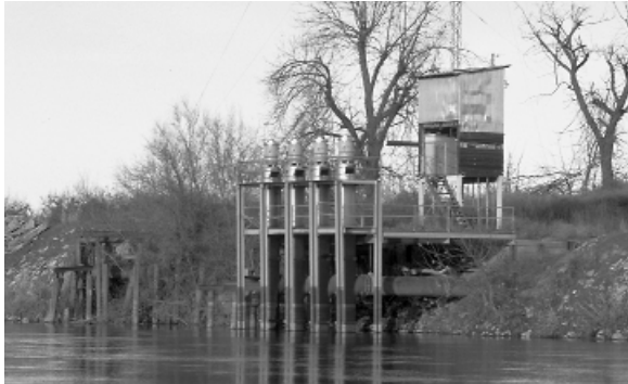
Major irrigation pumps taking water from the Sacramento River. (Photo: P. Gleick)
