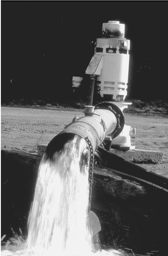
Groundwater pumps provide considerable water for California agriculture. For the most part, these pumps are not metered and groundwater use is not monitored, leading to overdraft in many regions. (Courtesy of DWR.)
