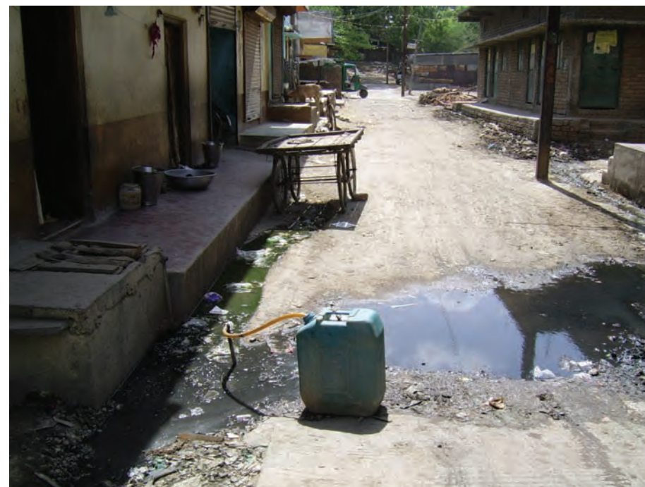
Drinking water being collected from a pipeline running through the open drain. © TARU
